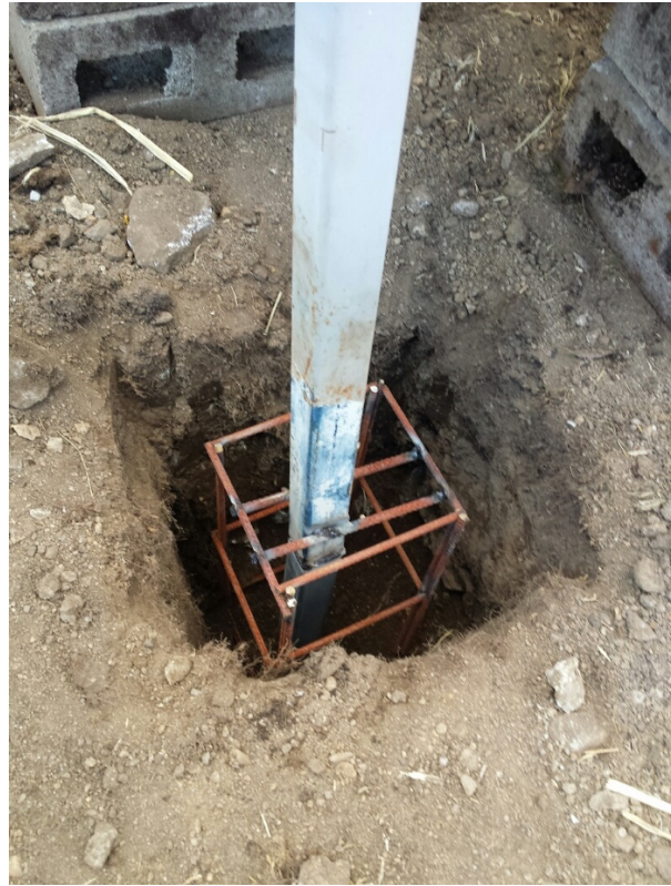
Typical footing excavation for Operators Hut
